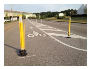
Some of you might have noticed that we are in the process of installing new traffic delineators along our bike lane in Munhall. Pictured below (in yellow) are two of our new rebounding delineators we recently installed by the Pump House. They are meant to help increase safety along East Waterfront Drive.
